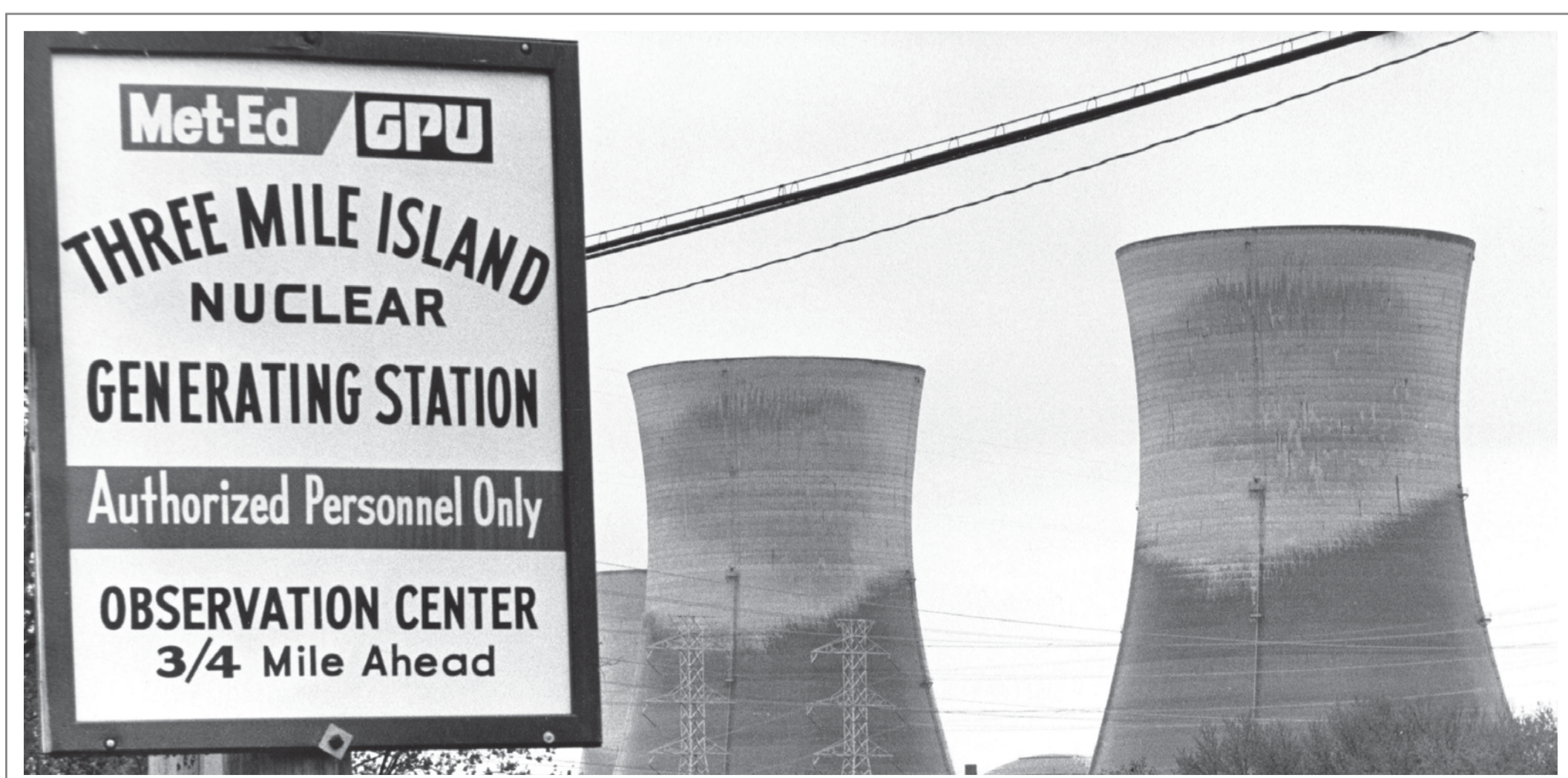
The Three Mile Island Nuclear Plant.
