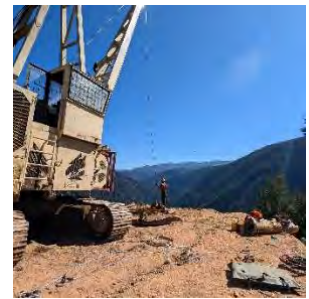
Figure 2. A rigging crew worker waits while coworkers set wire rope chokers on trees to be yarded up the hill on a cable logging operation with greater than 100% slope in north Idaho, August 2024.
