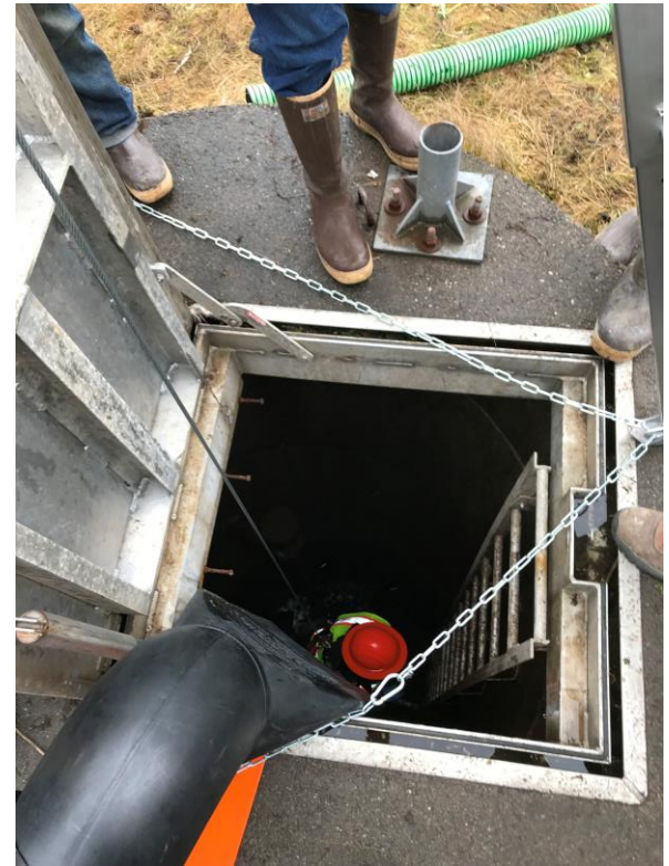
Angoon, AK – October, 2018 Lift station rehabilitation
