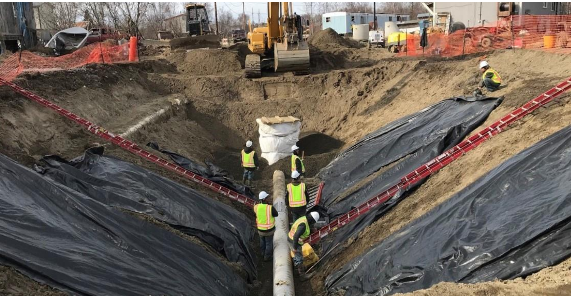
Lower Kalskag, 2018 sewer main construction
